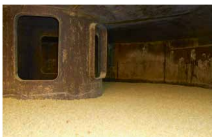
Fig. 3: Reactor bed of Quattro catalyst.
